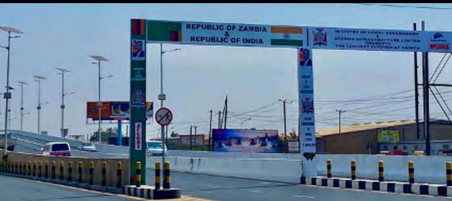
Flyover bridge on Kafue road as part of the Lusaka decongestion project. Infrastructure projects are said to be drivers of Zambia's external debt position.
