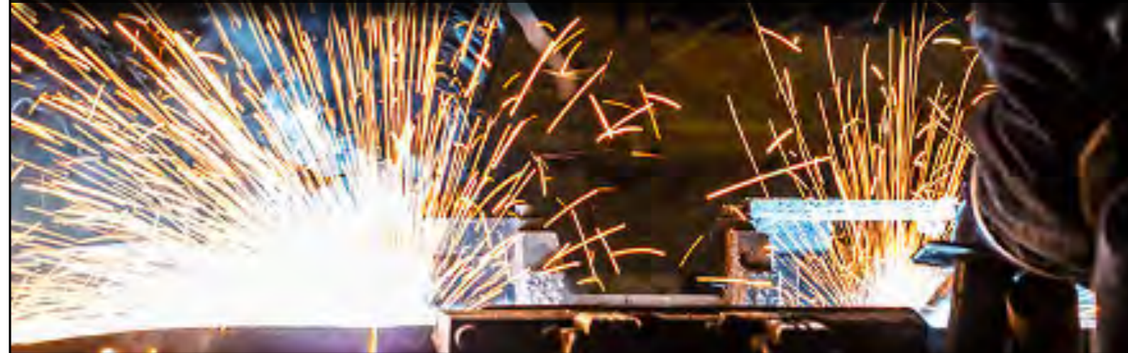
Welding activity on Zambia's Copperbelt Province.
